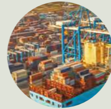
DP WORLD TERMINAL
